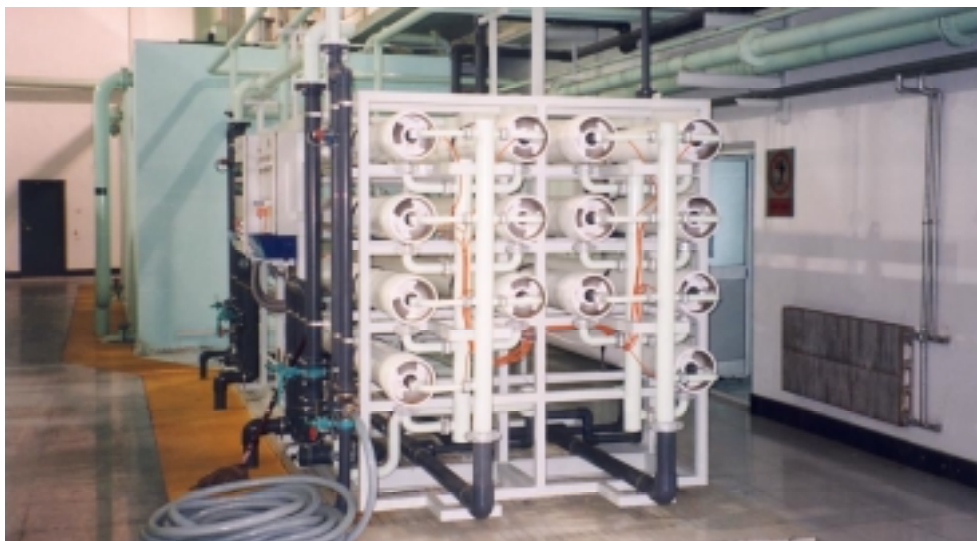
FILMTEC™ BW30-400 elements are used in the second-pass stage of the desalination process at the Huaneng Weihai Power Plant. (Photo courtesy of Huaneng Weihai Power Plant.)
